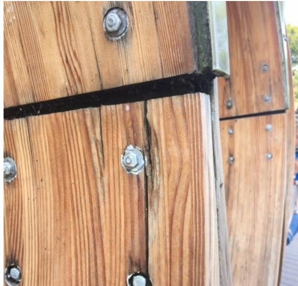
Figure 12. Splitting at Connections
