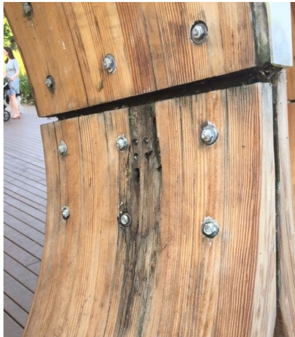
Figure 4. Wood Spalling at Grid C – East
