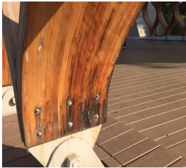
Figure 9. Dark staining at Grid J-West
