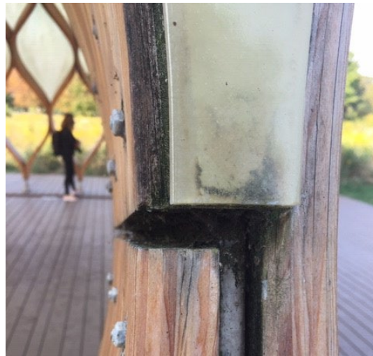
Figure 10. Chinking in Connection Joints
