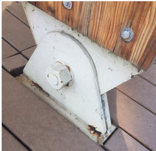
Figure 3. Visible Rust at Steel Base Connection
