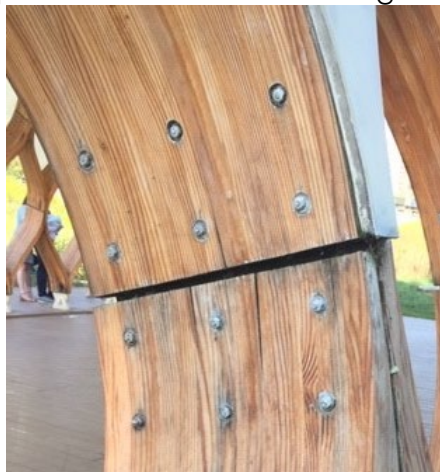
Figure 11. Thru-bolts at Typical Connections
