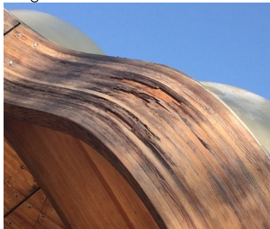
Figure 6. Wood Spalling at Southside (Southeast)
