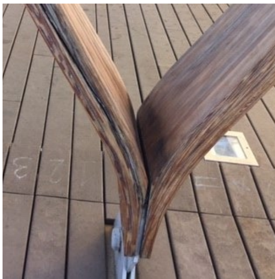
Figure 13. Missing Chinking at Base Connections
